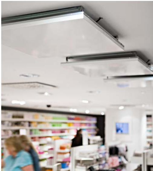
Mounting on the ceiling protects Thermocassette against damage.
